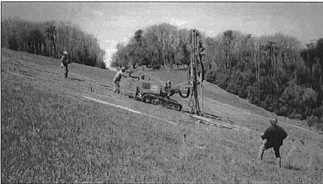
LMG grouting using 4 inch casing and rotary drill rig.
