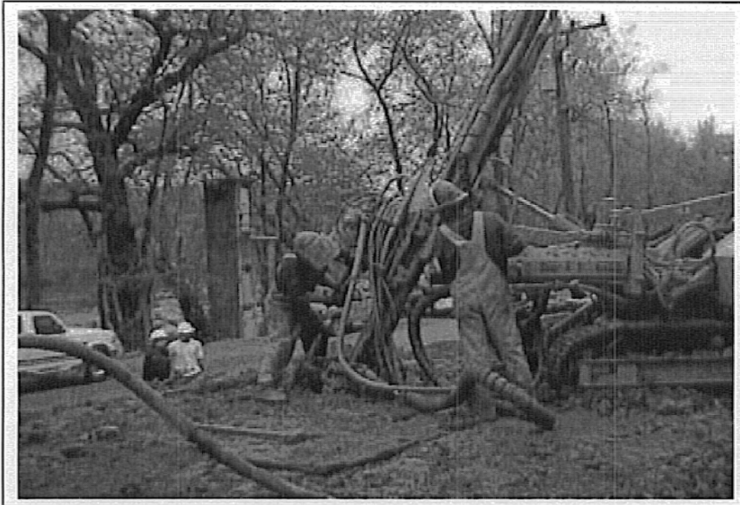
Grout hole drilling
