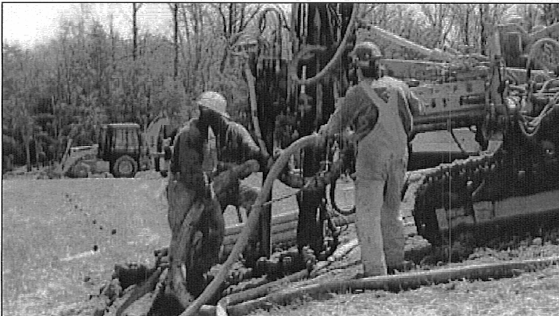
Grout injection to fill CMP conduit in dam.
